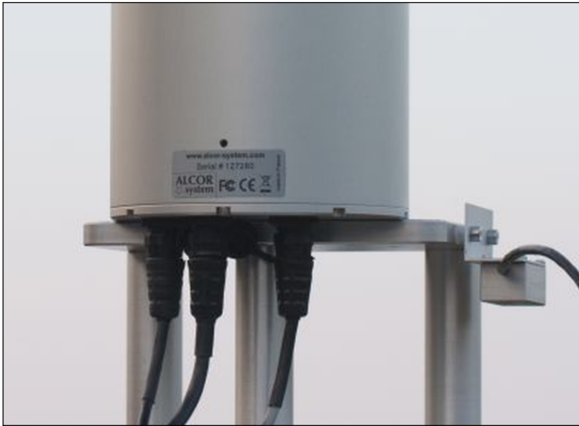
Fig. 24 Camera installed into a camera support
